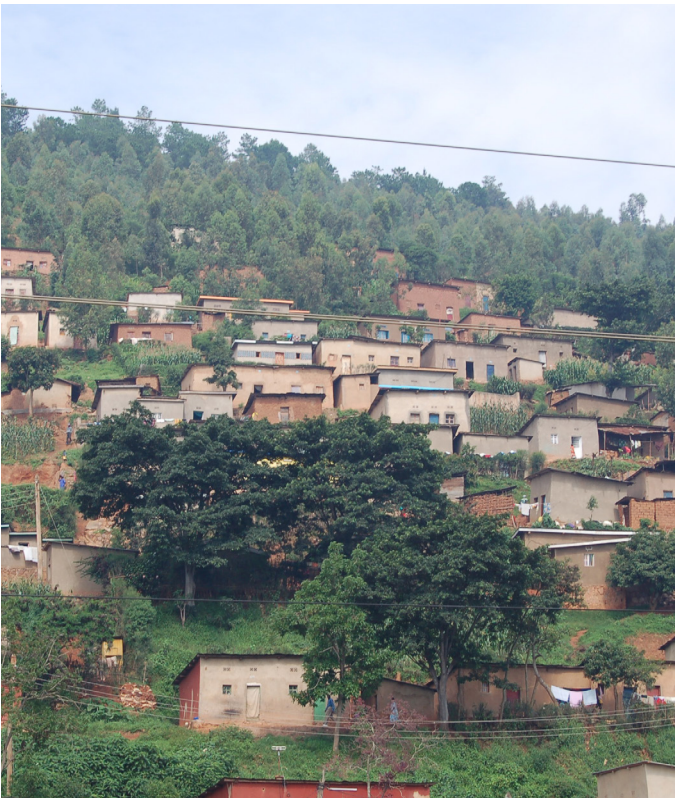
Houses on a hill slope, Rwanda
