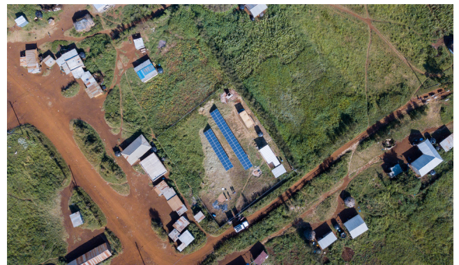
Aerial view of Marsabit County in Kenya © GIZ
